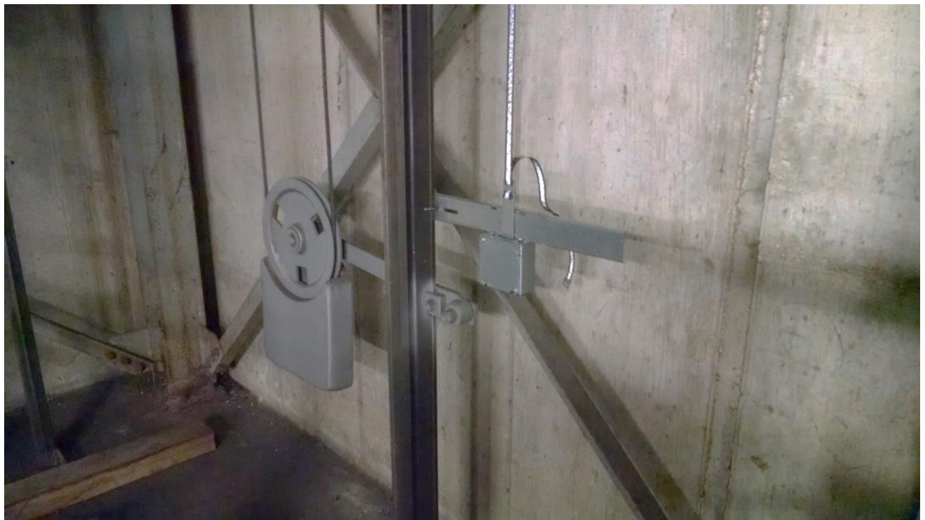
Figure 2-8: Encoded Tape Mounting – Bottom Bracket
