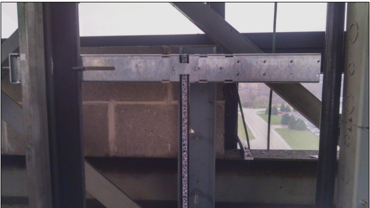
Figure 2-1: Encoded Tape Mounting – Top Bracket
